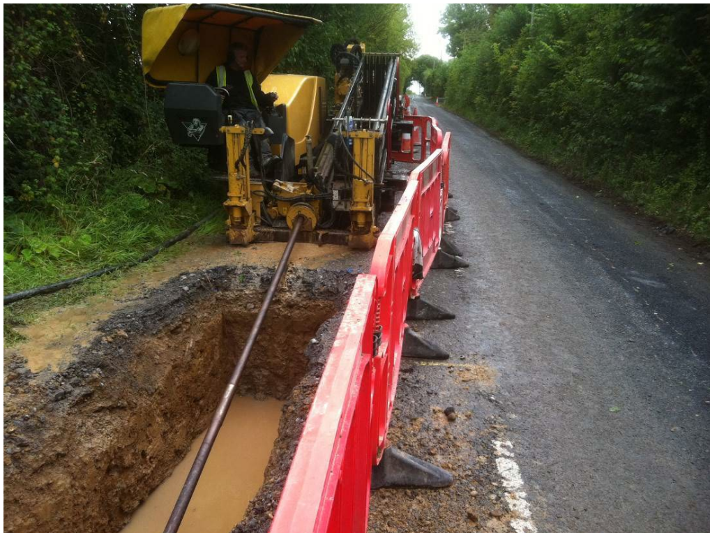
Figure 6: HDD rig set up on regional road.
