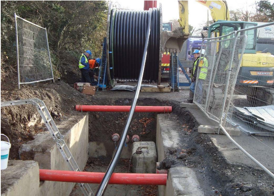
Figure 12 : HV cable pulling procedure (Standard drum set-up)
