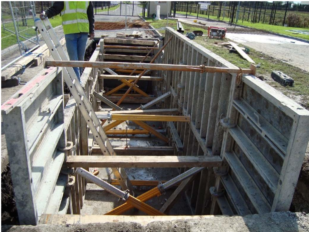
Figure 9 : Standard Joint Bay Under Construction (in-situ)
