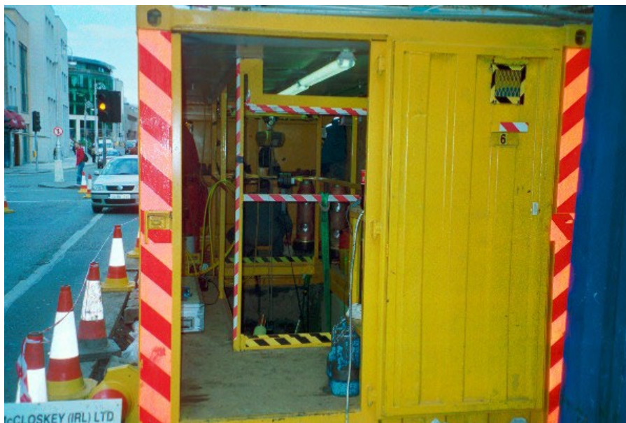
Figure 15 : HV cable jointing container
