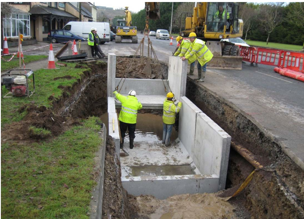
Figure 11 :Standard joint bay under construction (pre-cast)
