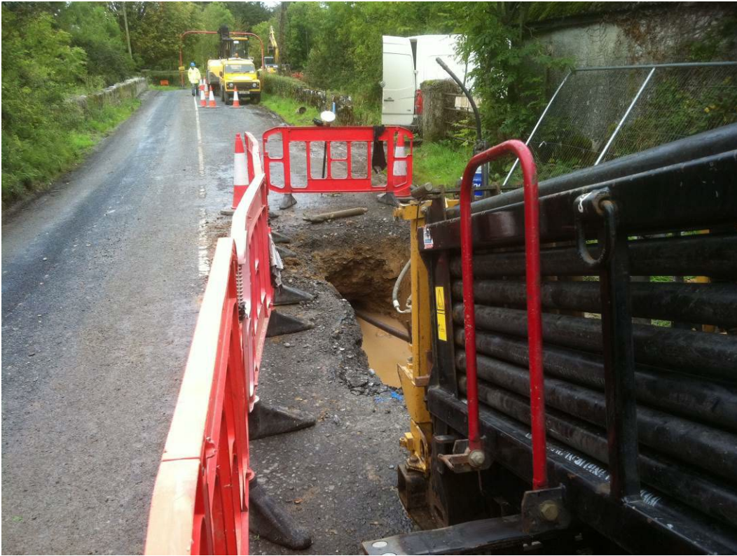
Figure 7: Standard HDD site on local road where HDD was used to go underneath a bridge (bridge parapet walls visible)
