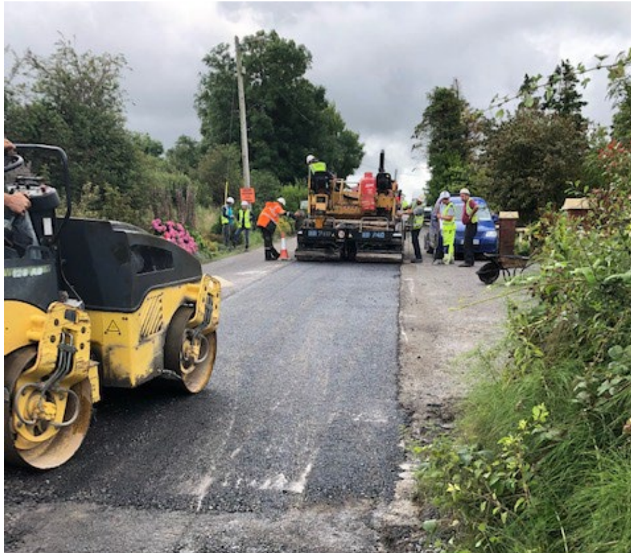
Figure 2 : Permanent Reinstatement of road surface over trench
